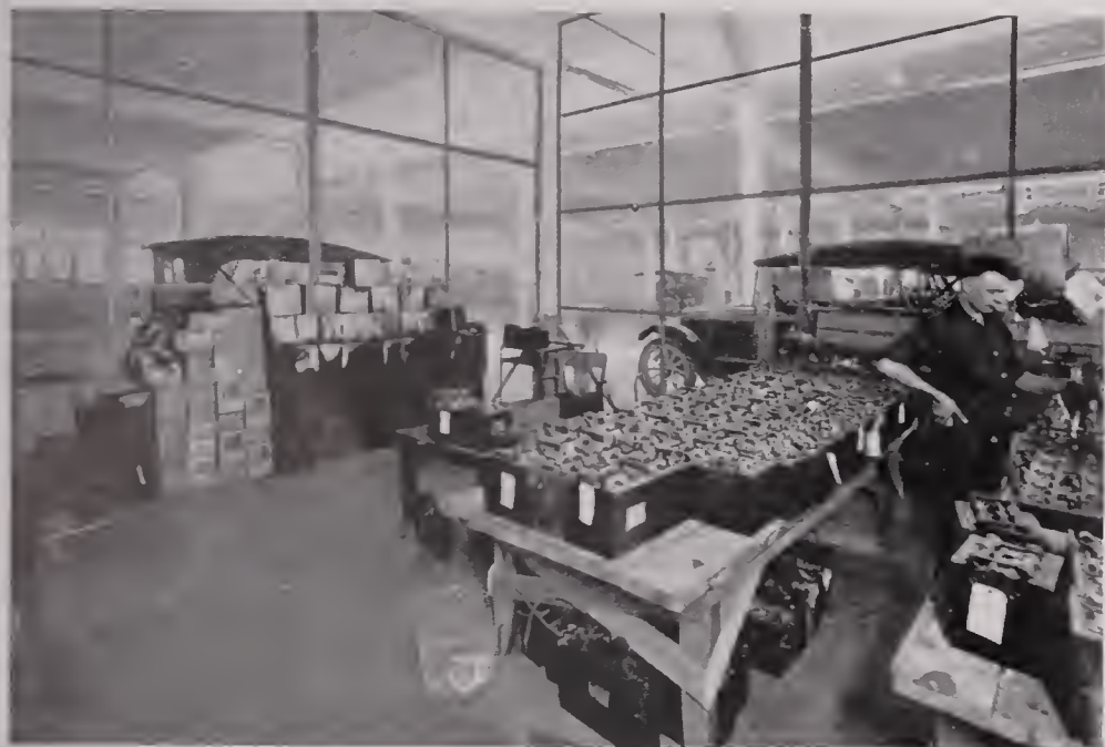
BATTERY TESTING AND CHARGING DEPARTMENT
